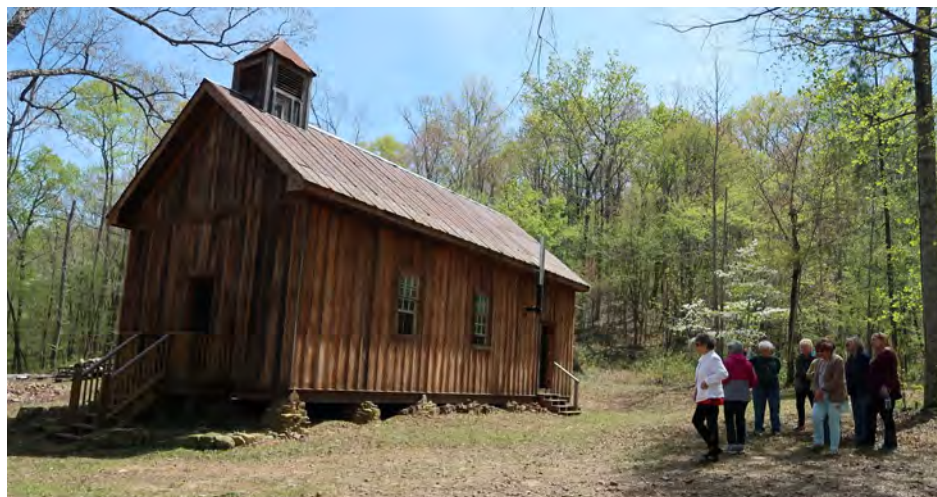
GLENDALE CHAPEL AFTER RESTORATION
